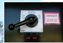
Multi-Voltage Selector Switch
